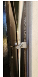
Example of D-ring over hook
